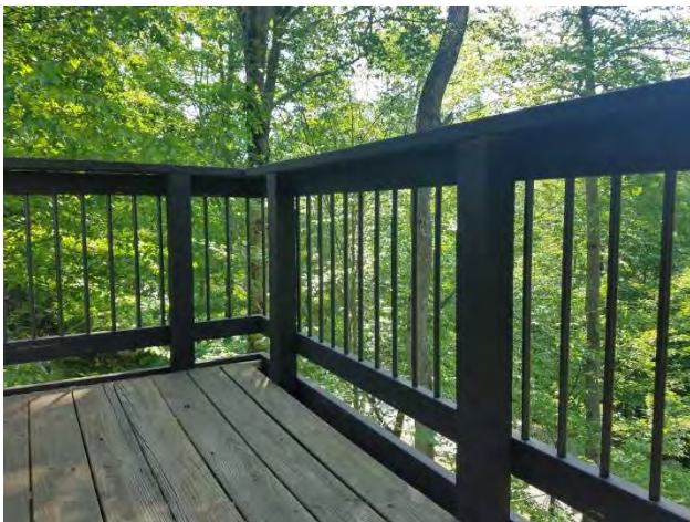
Figure 3 Image of alternate stair rail
