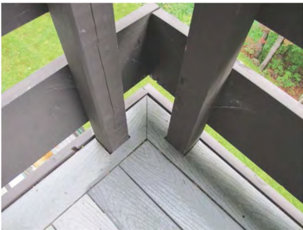
Figure 1 Decking notched around posts flush with lower 2x12
