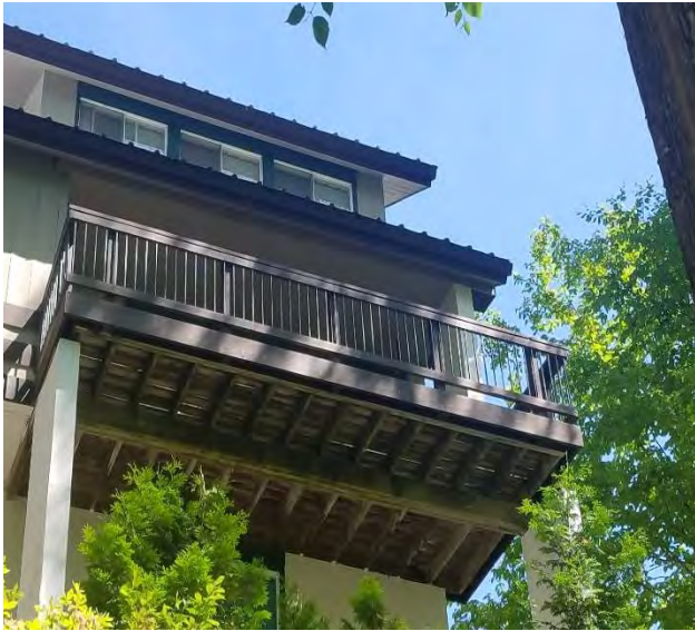
Figure 2 Image of alternate deck rail
