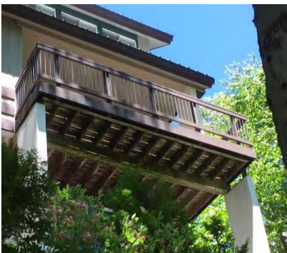
Deck rail at 90 Coolidge Falls Road
