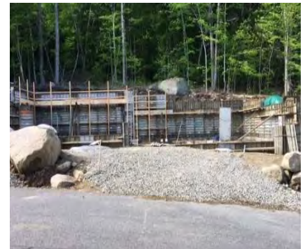
Foundation poured on Highview
